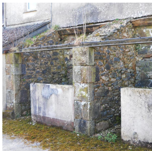
Fig. 16 - stone buttresses supporting shippon wall.
