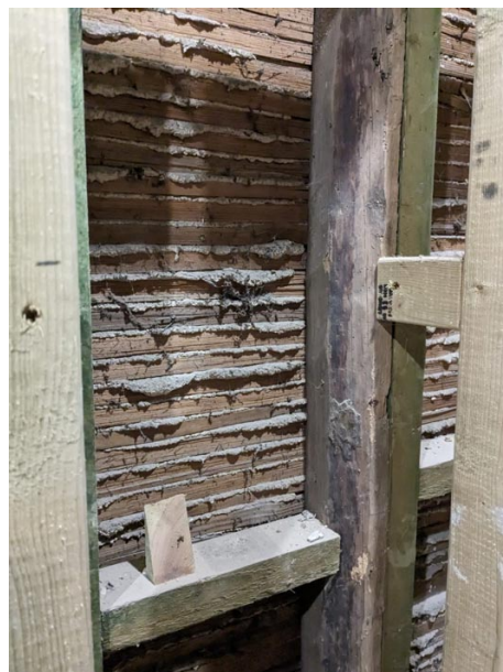
Fig. 15 - lath and plaster finishing of wall between parlour and cross-passage.
