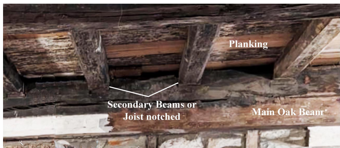
Fig. 11 - smaller beams notched into major oak beams to which second floor planking was attached.
