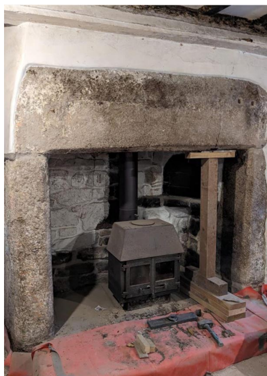
Fig. 13 – fireplace on ground level
