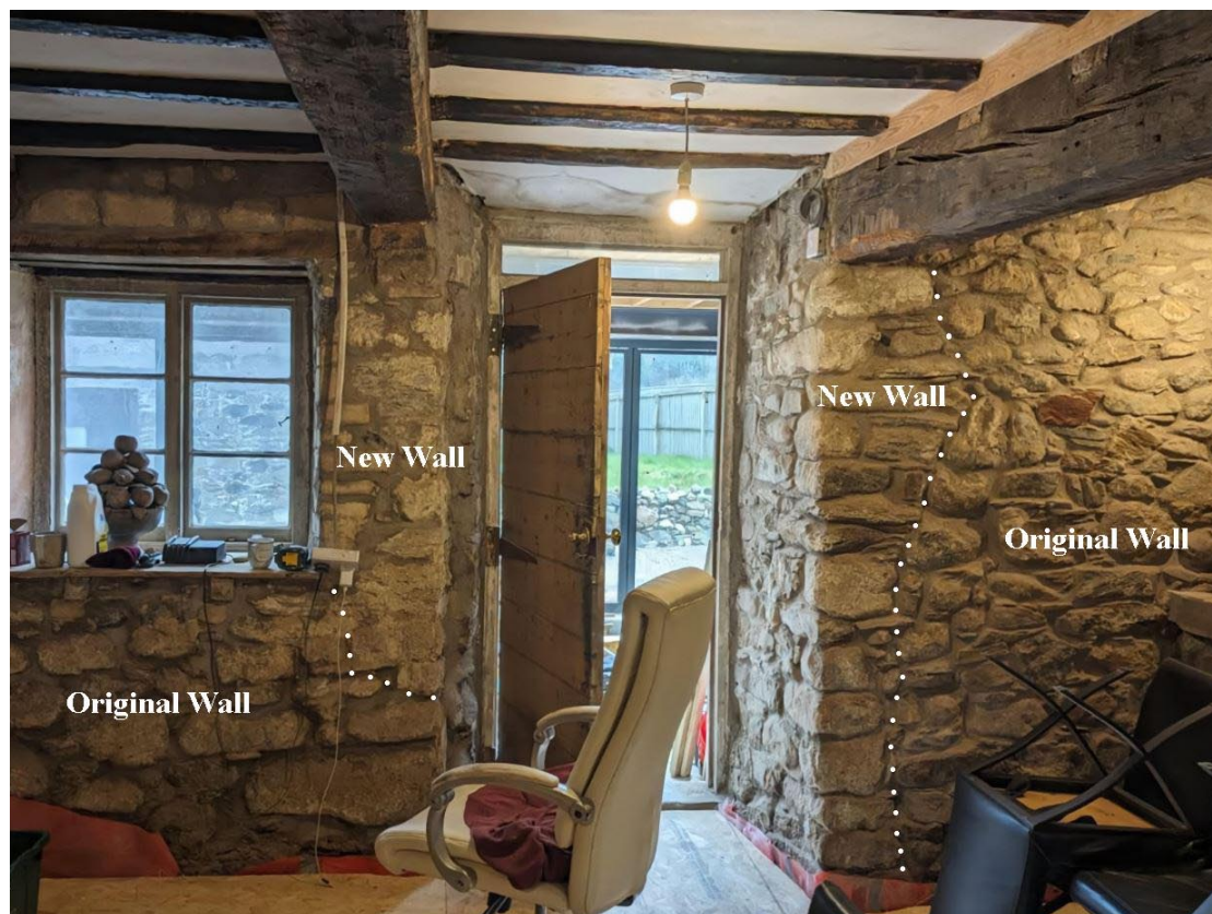
Fig. 10 - part of original exterior wall, modified to accept horizontal beams for second floor construction; lower wall under window and main wall to right of door made from uncut stone generally laid 1 over 2 and 2 over 1; window framing set on wood members set into original wall; wall between window and door and to the right of the door partially rebuilt with masonry or cut stone to hold beam; wood headers installed over window opening to support masonry.
