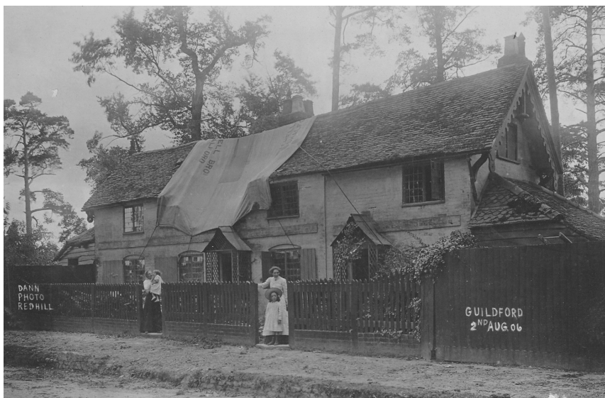
Photograph 2: Storm damaged cottage
