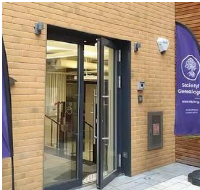
Figure 1b. SoG premises, 2024
