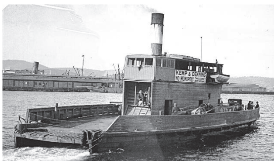
Centenary history of Kemp & Denning Limited, 1902 - 2002 by A L Graeme-Evans.
