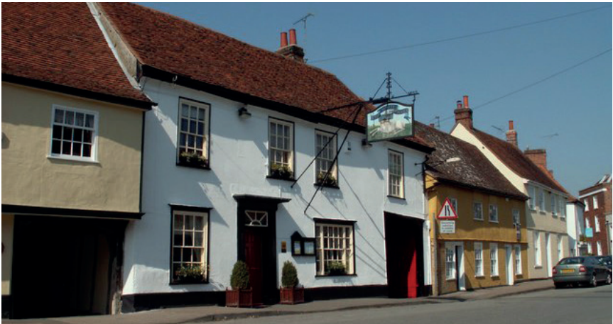
The White Hart, High Street, Nayland, showing carriage entrance (Robert Edwards / The White Hart inn, High Street, Nayland / CC BY-SA 2.0)
