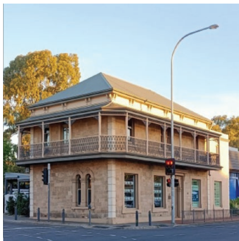
Waverley House, originally home of the MALLEN family, on the corner of Belair Road and Princes Road, 2025 (Image courtesy of the author)
