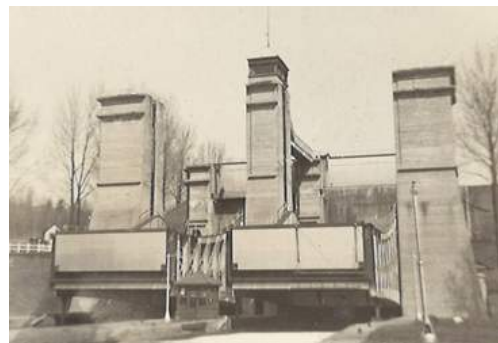
Below: Fig. 21 - Lift locks at 220 Hunter Street East
