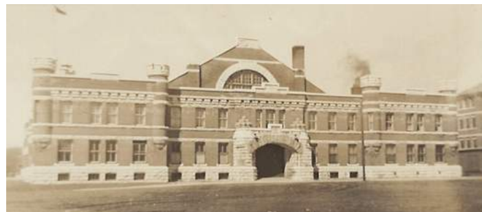
Below: Fig. 16 - Drill Hall/Armory at 220 Murray Street
