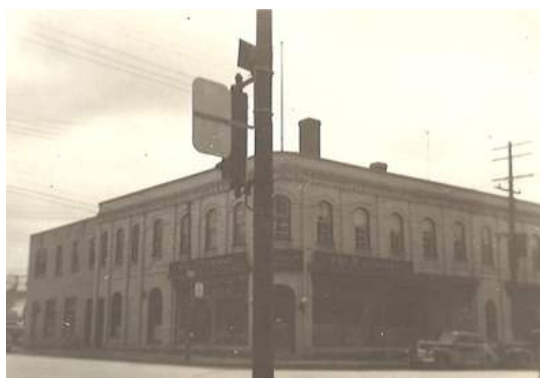
Above: Fig. 20 - The Peterborough Examiner Building, home to the newspaper for a time
