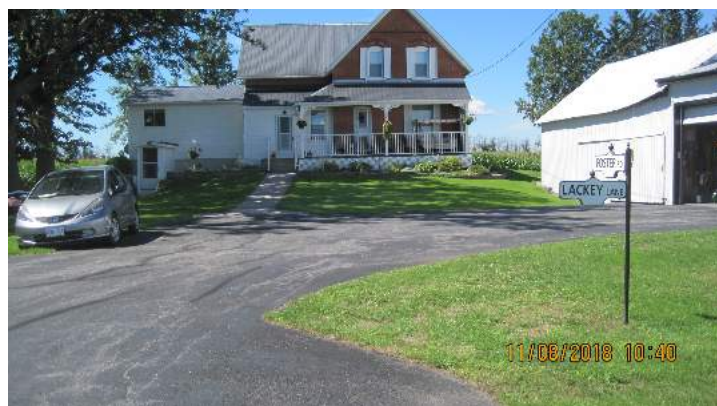
The 1897 brick house built on the SE Pt. Lot 25, Con. 5, Goulbourn Twp. (8/11/2018)
