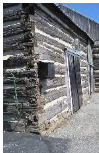
A side view of the old-growth squared Cedar logs of the pioneer barns. (8/11/2018)
