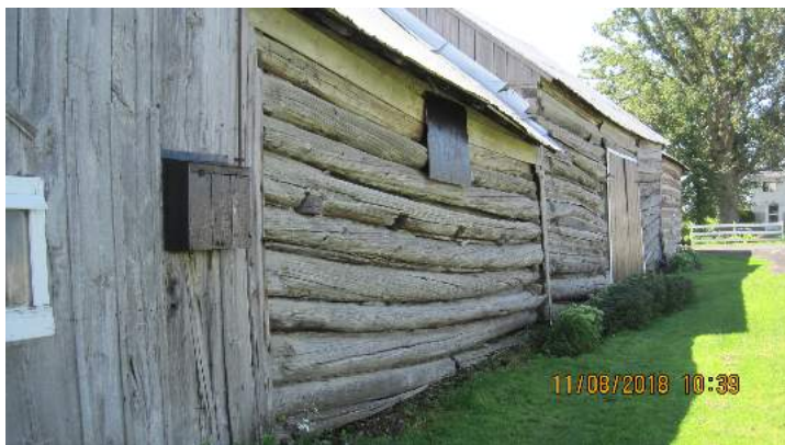
A side view of the old-growth squared Cedar logs of the pioneer barns. (8/11/2018)
