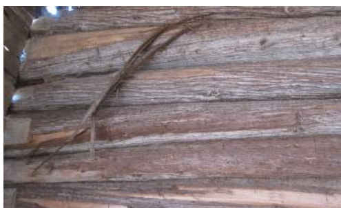
A side view of the old-growth squared Cedar logs of the pioneer barns. (8/11/2018)
