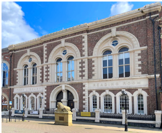
Mechanics Institute, South Shields
