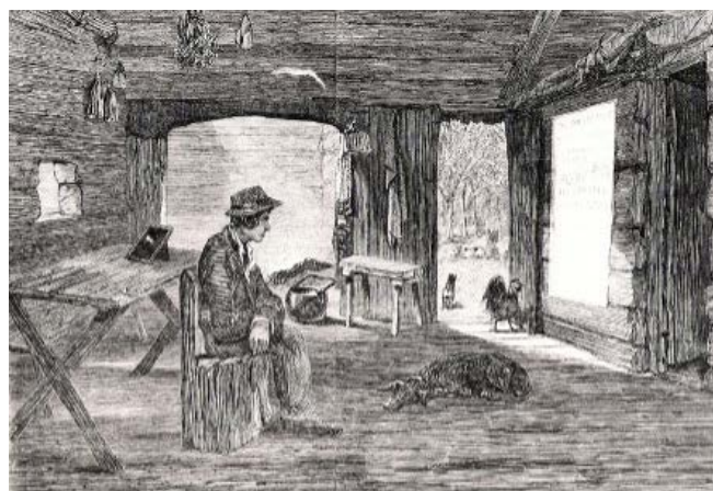
Slab House Interior 1849
