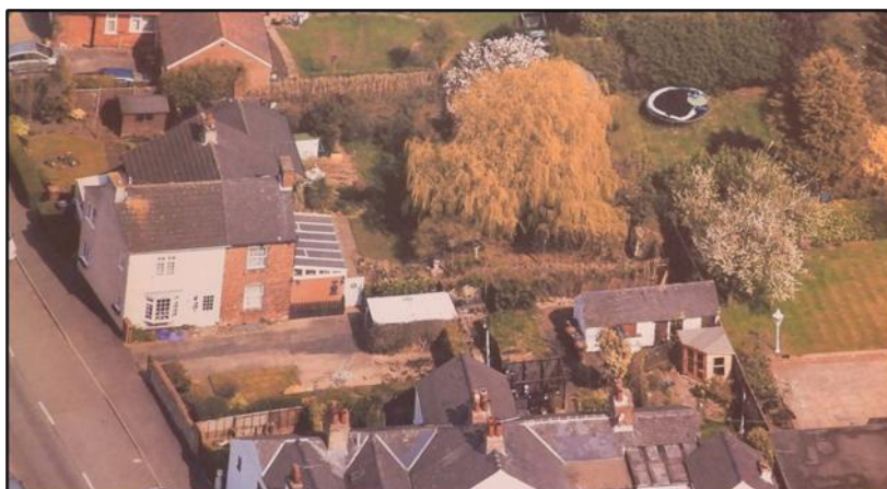
Bird's-eye view of No's 94 and 96
