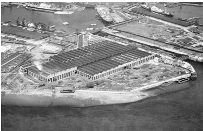
HARLAND AND WOLFF, NORTH WOOLWICH
