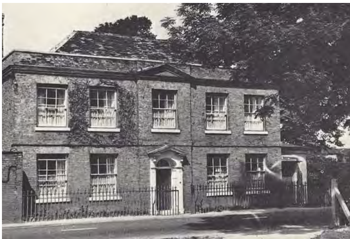
ASHBROOKS DAGENHAM, AN 18TH CENTURY HOUSE WHICH WOULD HAVE BEEN SUBJECT TO THE WINDOW TAX. IT WAS ORIGINALLY CALLED SPARKS.
