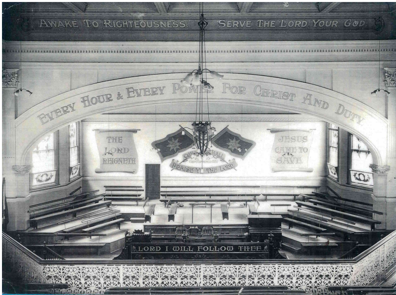
Interior Old Salvation Army Congress Hall, ca 1912, Goulburn St. (photo: courtesy of The Salvation Army Museum Australia)
