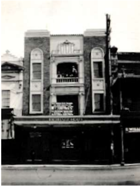
Newly Renovated Exchange Hotel 1930 (photo: Lunney family album)
