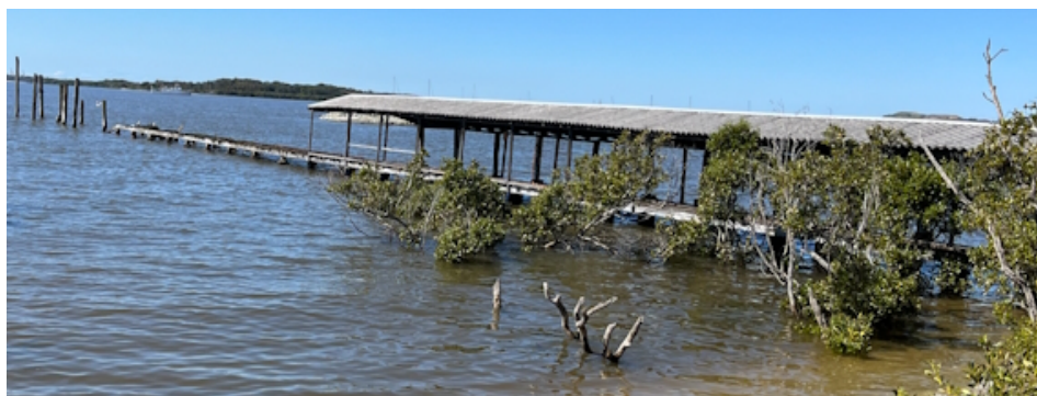
Timber Pile Jetty (photo: Pat Fearnley)
