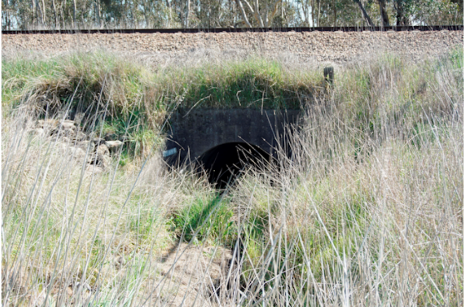
Upstream side of the rebuilt culvert showing the current drainage tunnel in 2023 (photo: Doug Butler , licensed under the Creative Commons Attribution-Share Alike 4.0 International license)
