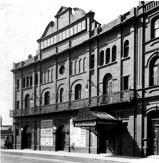
This shows the brick construction, before trams were introduced
