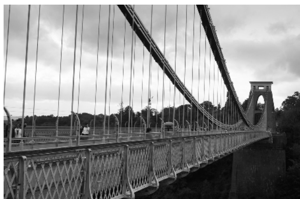
Clifton suspension bridge
