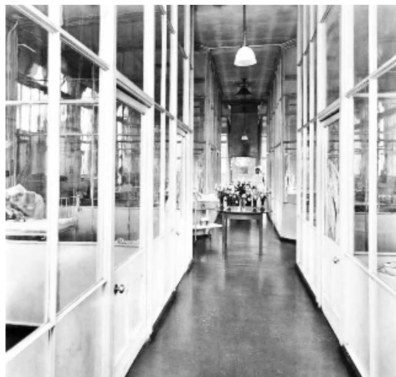
Isolation cubicles in Eastern Hospital treatment of infectious patients Image courtesy of George English
