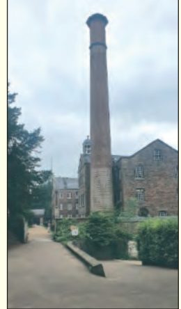
The Mill chimney.
