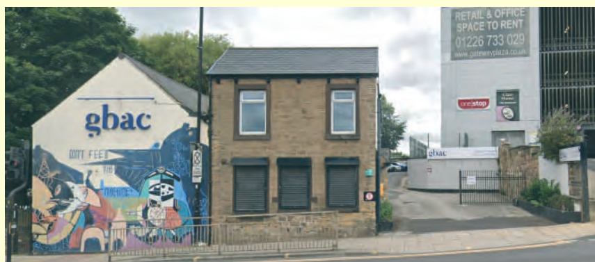
Street View 2024; new roofs, new windows, but old stonework?
