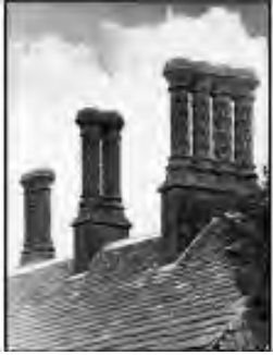
Elizabethan Chimneys (courtesy MDT)
