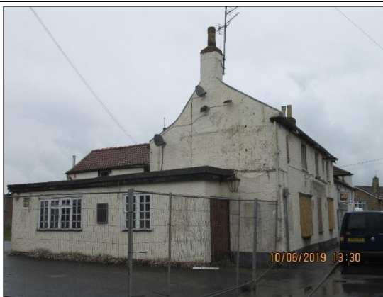
Sun Inn, Skirlaugh, seen in 2019 after demolition was halted
