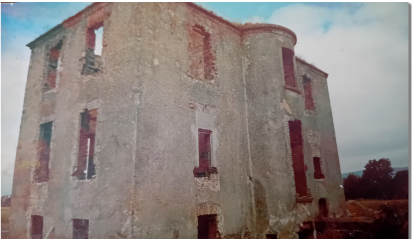
The damaged original Killonerry farmhouse, pictured here prior to its restoration (photo courtesy Susan O' Mahoney).
