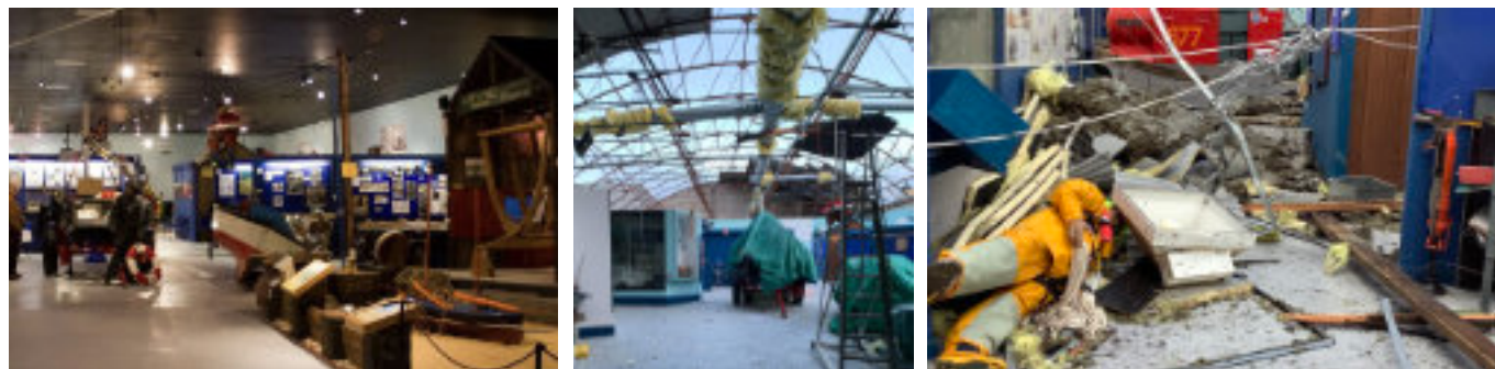
Before (left) and after (middle and right) pictures of the Fraserburgh Heritage Centre, showing the damage caused by Storm Arwen. Photos: Fraserburgh Heritage Centre
