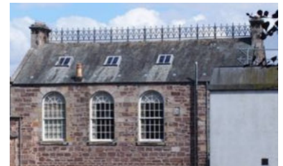
Prison roof from the back
