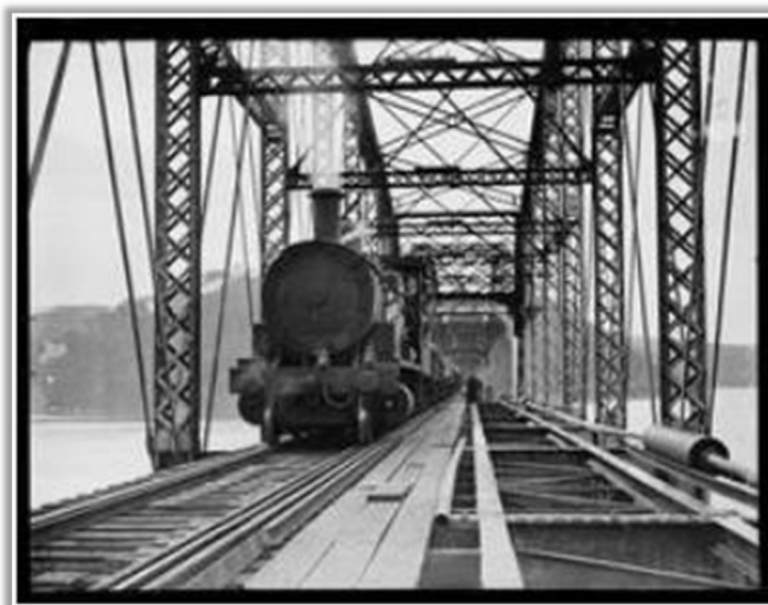
Train crossing the Hawkesbury Bridge
