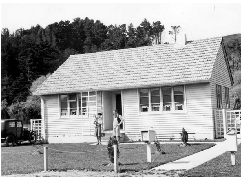
Typical New Zealand house 1920-1930
