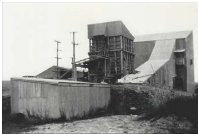
Rear of Waitotara Lime Works.
