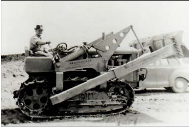
Charlie Hodgetts on the first bulldozer purchased by the Waitotara Lime Company.
