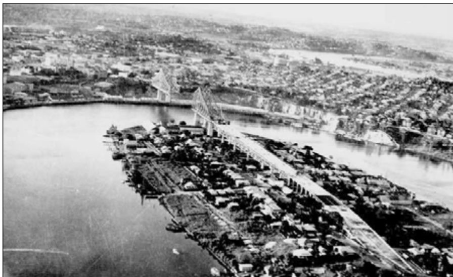
Figure 3. Brisbane River and Story Bridge, 1939. Aerial view of Kangaroo Point and the Brisbane River, including the incomplete Story Bridge under construction. John Oxley Library, State Library of Queensland. https://hdl.handle.net/10462/deriv/136470
