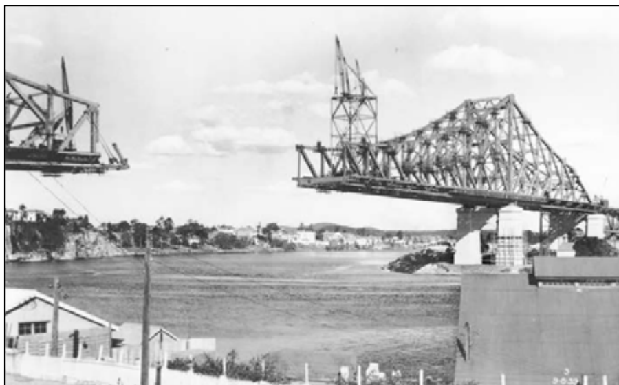
Figure 4. Brisbane's Story Bridge under construction, 1939, viewed from the north side. John Oxley Library, State Library of Queensland. https://hdl.handle.net/10462/deriv/94436
