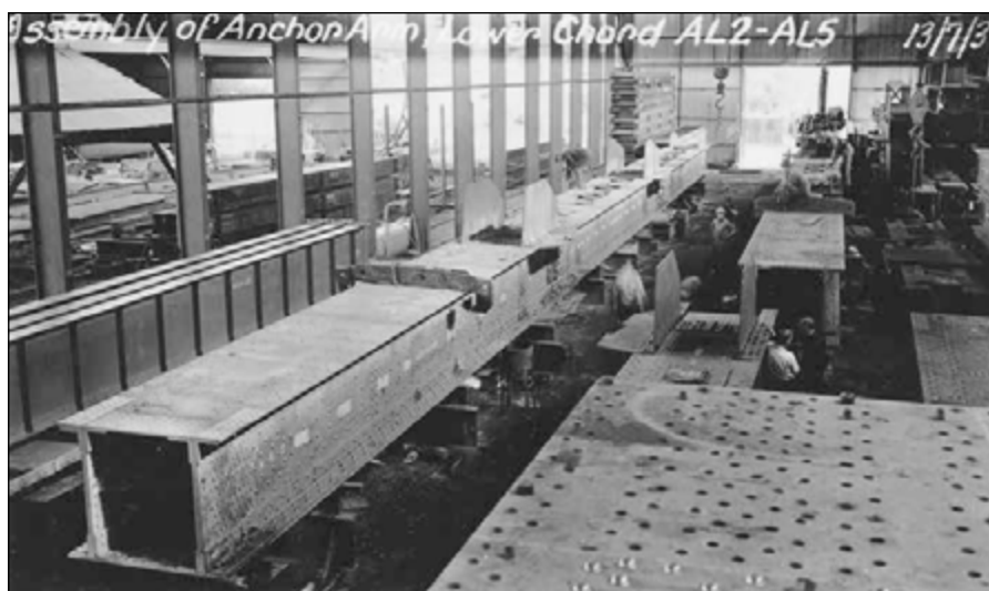
Figure 2. 'Assembly of Anchor Arm, Lower Chord AL2-AL5 13/7/37', showing steelwork with some of the 1.25 million rivets. Story Bridge Construction Photograph Album (0001-0185). John Oxley Library, State Library of Queensland. http://hdl.handle.net/10462/deriv/241925
