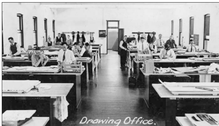
Figure 1. Brisbane River Bridge Board. 'Drawing Office'. Lauren McDonald on left hand side, fourth from the front. John Oxley Library. State Library of Queensland. http://hdl.handle.net/10462/deriv/241906
