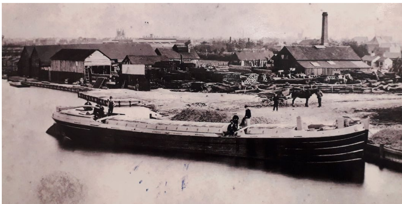
Barge building sheds of R Talbot & Sons at Caversham c1876 (courtesy of Reading Local Studies Illustration Collection)
