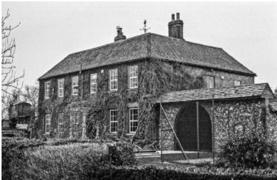
The much-altered front facade of Littlestoke Manor
