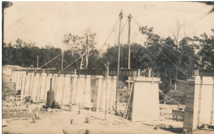
Glassford Creek Railway bridge under construction
